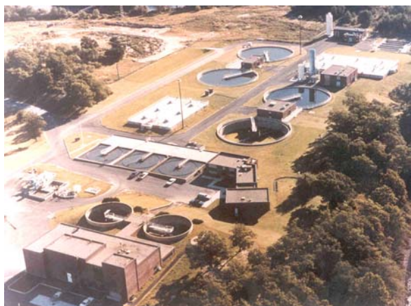
Aerial View of Taunton Wastewater Facility Before DBO
