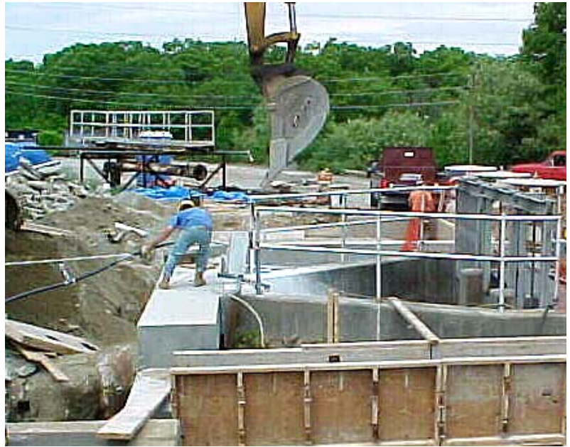
DBO Contract Construction of the New Headworks
